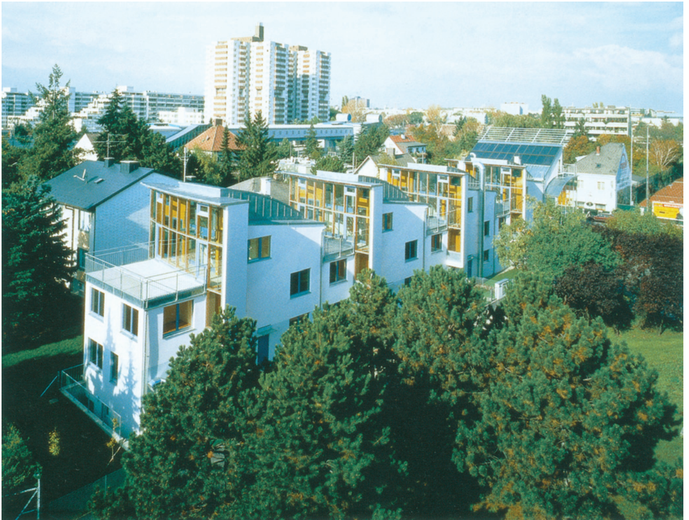
1.13. Professor Georg Reinberg's solar development in Sagedergasse, Vienna, making imaginative use of the building form to optimise the solar potential of the site (Reinberg, 1996).
