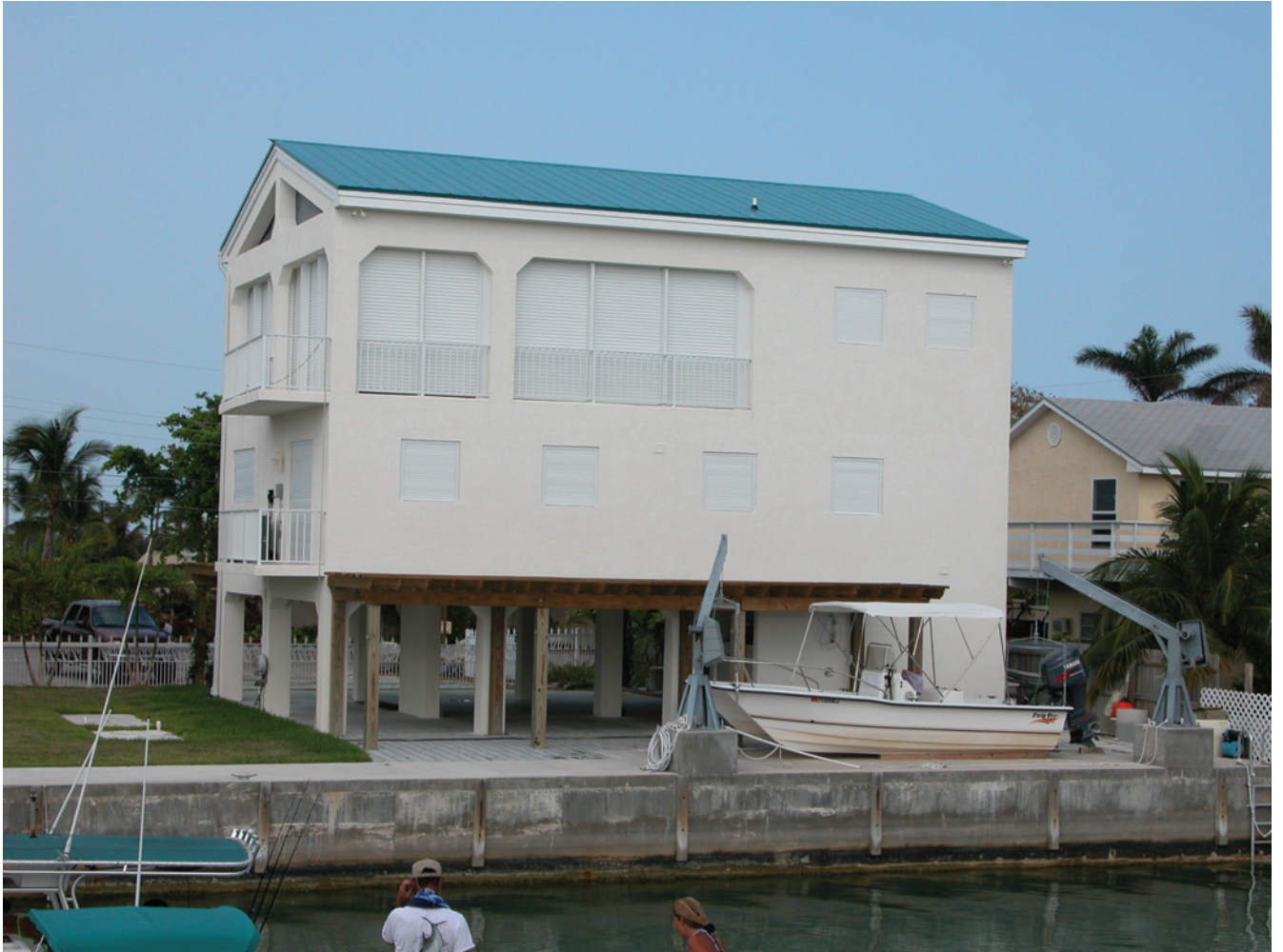
Porpoise Point Ecohouse, designed by Stephanie Thomas.
