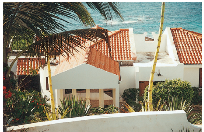
CS 16.12. Before Hurricane Lenny. Remodelled after Hurricane Luis with a new protected entry and roof tiles glued, screwed and cemented. By David Morrison.
